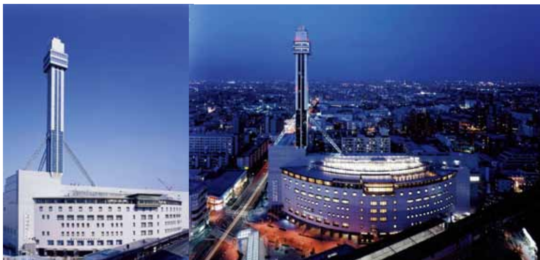
Tower Hall Funabori
